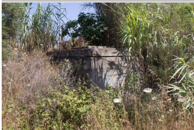
Cisterna in c.a.
